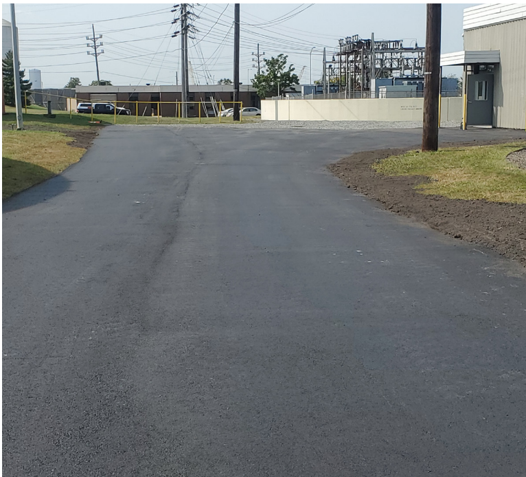
Completed paving project
