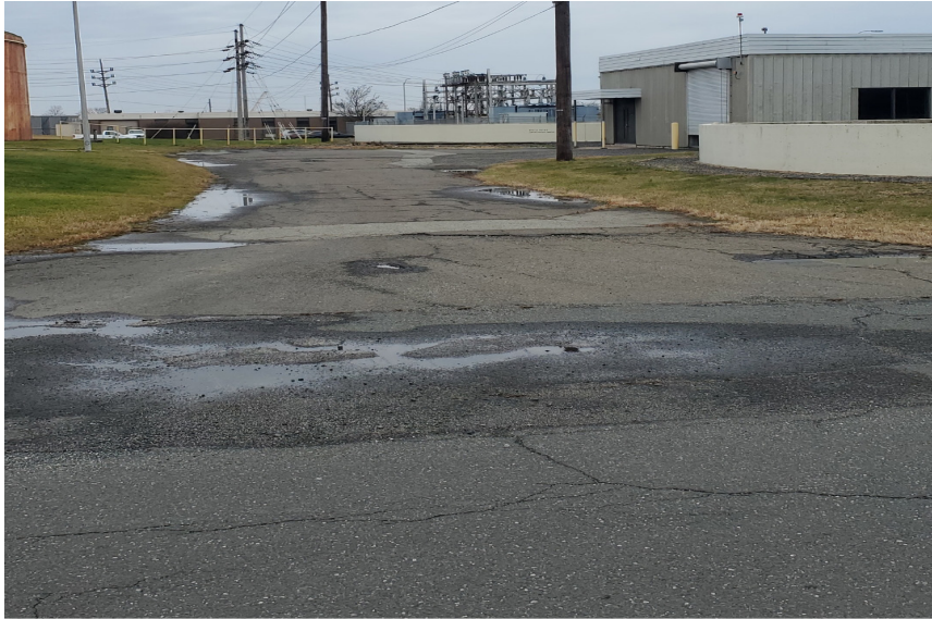
Road prior to paving
