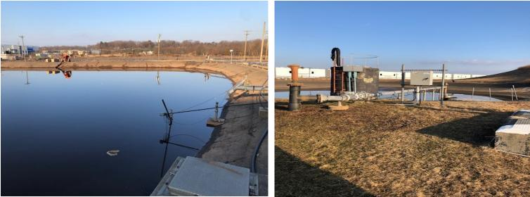
The perimeter of the Middlesex County Landfill contains four paved pond areas that collect and pump stormwater, that may have had contact with solid waste, into the Landfill's Leachate Collection System. Currently, each pond has a single pump system. The proposed upgrade will include a duplex pump system, new electric and piping.
