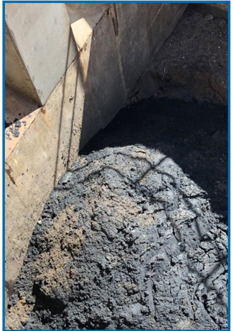
Grit Piled for Removal
