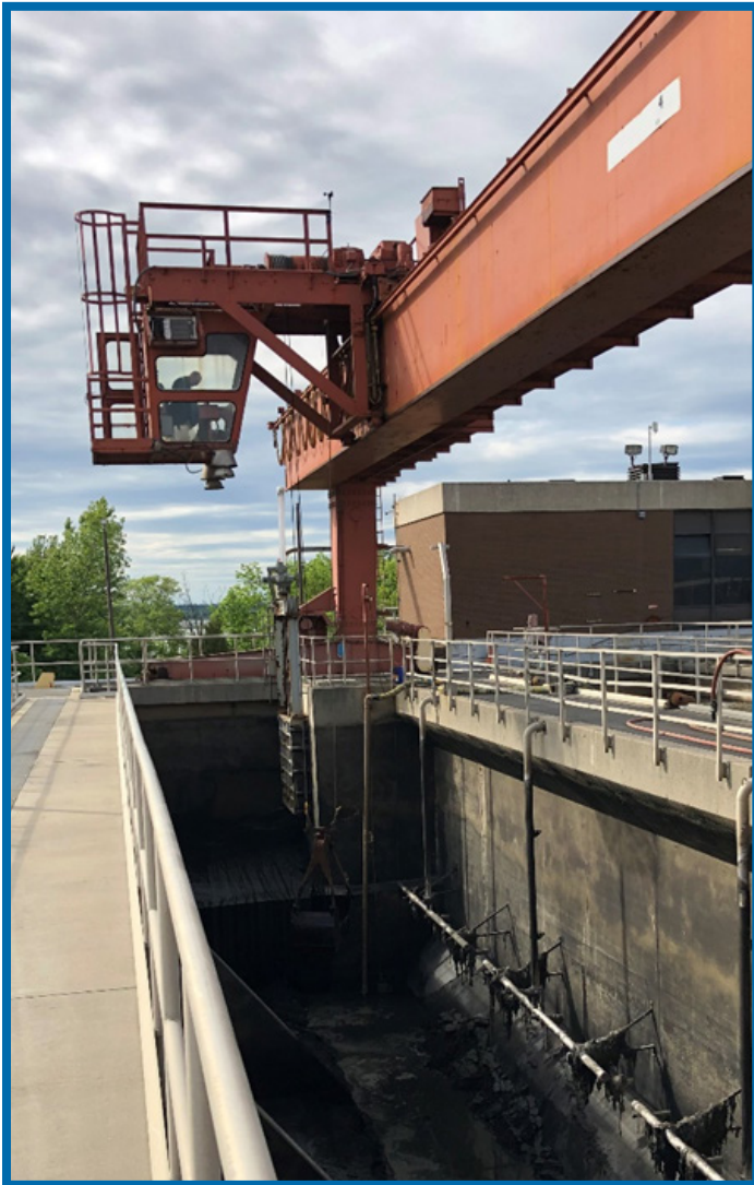
Greg Soroka Removing Grit with Gantry Crane
